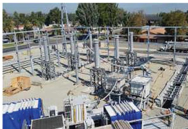
Setup of four RTS reactors.
