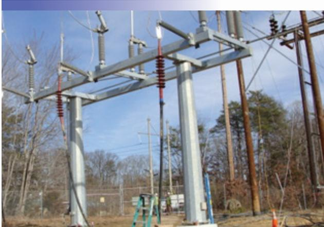
*Temporary cables enable bypassing sections of substation buses for maintenance.*
